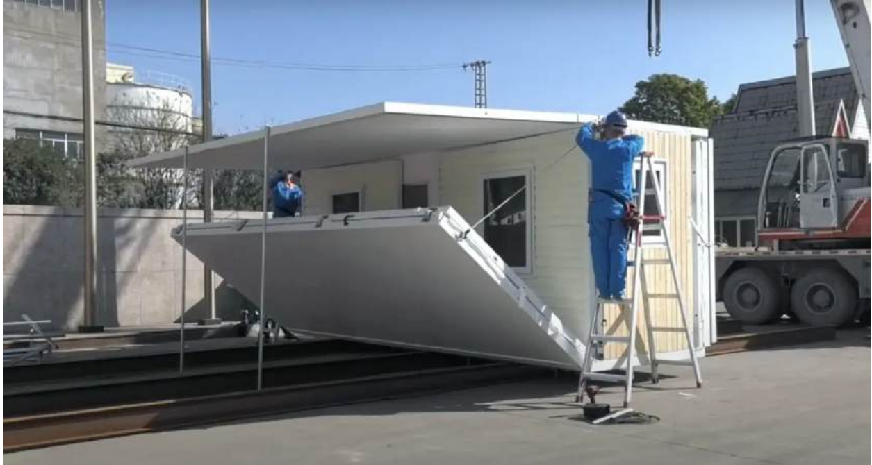
Two builders "unfold" a unit on site. Hapi Homes/YouTube
